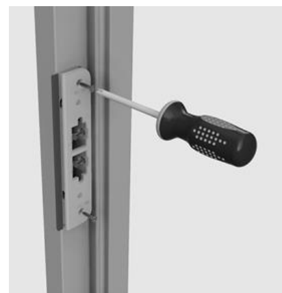
Figure 3 – Mounting the strike plate
